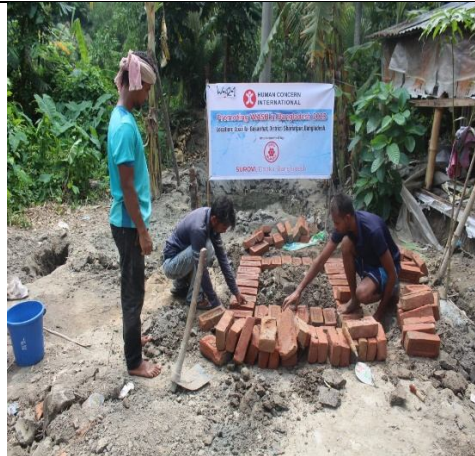
Constructing platform and pump house
